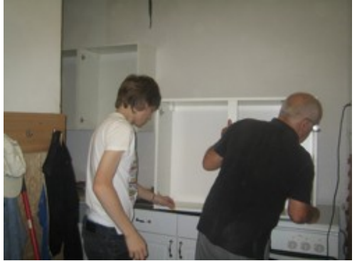
Colin and Luke at work on the new kitchen cupboards.
